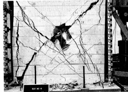
Shear failure mode (Courtesy of B. Shing)
